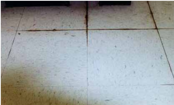
Moisture and high pH values dissolve adhesives ...
