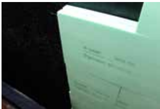
Insulation boards can be easily attached with two-component KÖSTER PMBCs. It is important that the insulation boards are fully bonded.
