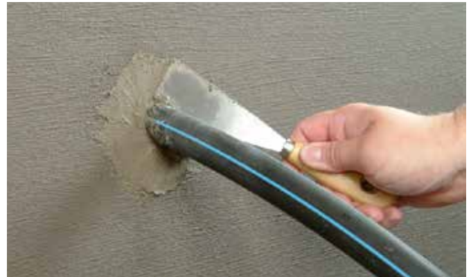
In order to protect the waterproofing and provide mechanical support, the area around the pipe or cable is plugged with KÖSTER KB-Fix 5.
