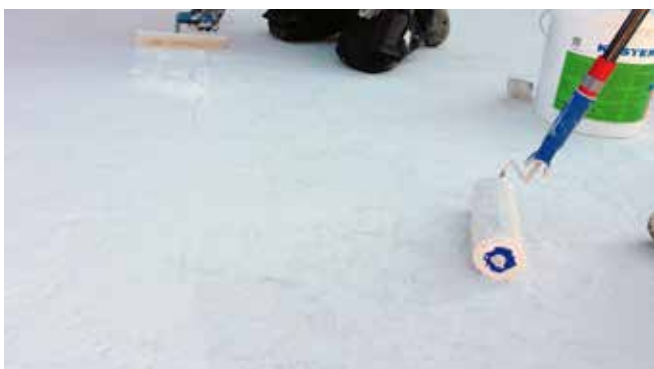
Application of the second layer of KÖSTER 21
