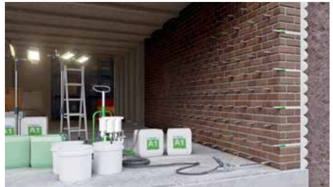
Curtain Injection of Masonry
