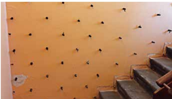
Injection into Concrete
