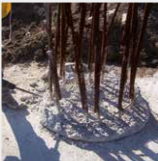
Removing protrusions, cleaning the pile head.
