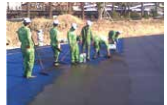
Waterproofing with KÖSTER Deuxan 2C
