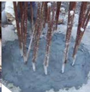
Installing a fillet and smoothing the area with KÖSTER WP Mortar.
