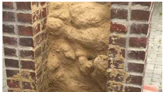
Curtain Injection (rear view)
