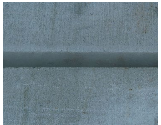
Cleaned joint flanks
